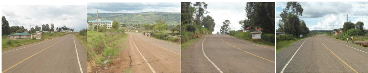
Photo 2.8: Reconstructed Town Roads.
