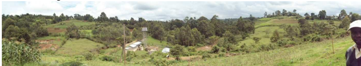
Photo 2.3: Mogombet Water Intake and Treatment Works
